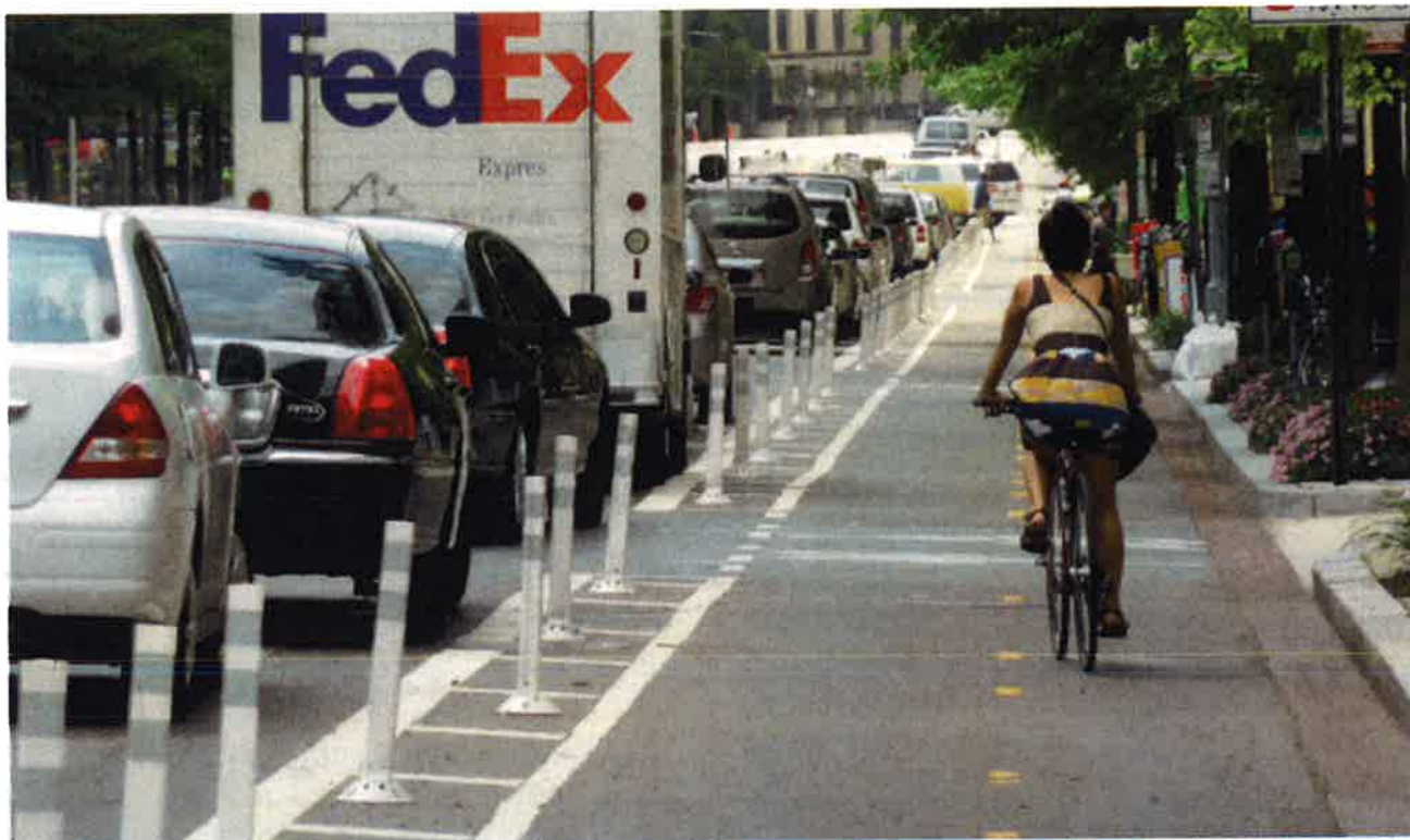
Cycle tracks can be designed to be two-way facilities on a one-way street. Signage and pavement markings are provided at driveway crossings to alert drivers to the presence of two-way bicycle cross traffic.
