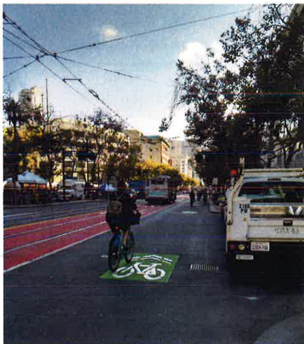
Green-backed priority shared lane markings are more visible and spaced more closely than normal sharrows.
