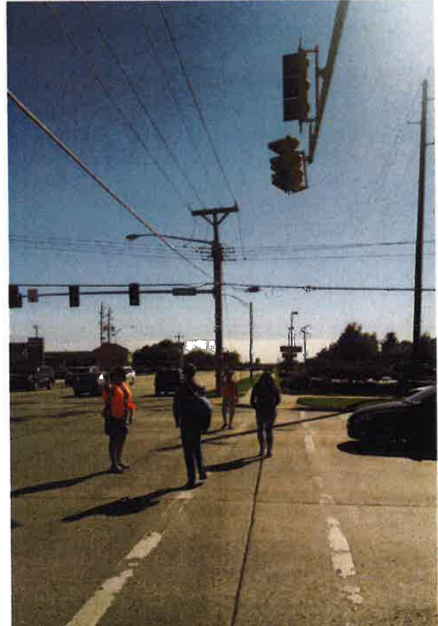
Standard crosswalks consisting of two parallel white lines are less visible to drivers than zebra or ladder designs that include wide white stripes perpendicular to the road edge. Stop bars are also needed at intersections to direct drivers to stop at a greater distance from the crosswalk, making it less likely they will block a pedestrian's path of travel.
