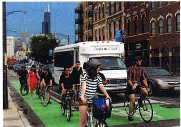
Bicyclists wait in a bike box in Chicago, which increases their visibility and reduces their signal delay.
