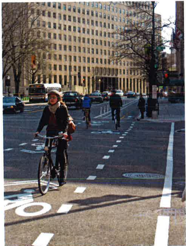
Striping bike facilities through intersections highlights the bicyclist's path of travel.
