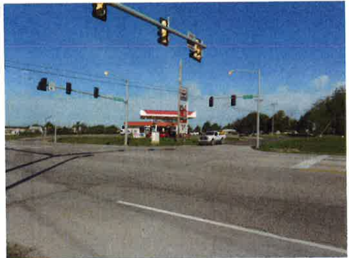
Lack of crosswalks and ramps at intersection
