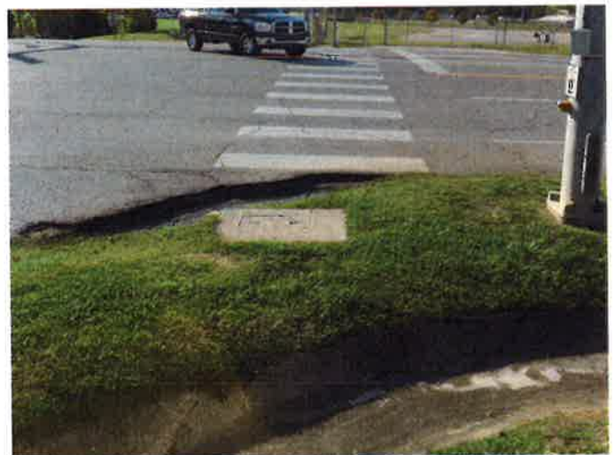
No ADA compliance or connection to sidewalks
