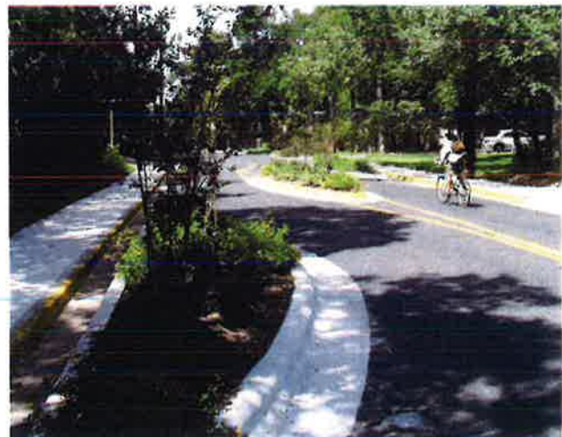
Chicanes divert traffic horizontally and may be designed to create a one-lane street that necessitates driver yielding.
