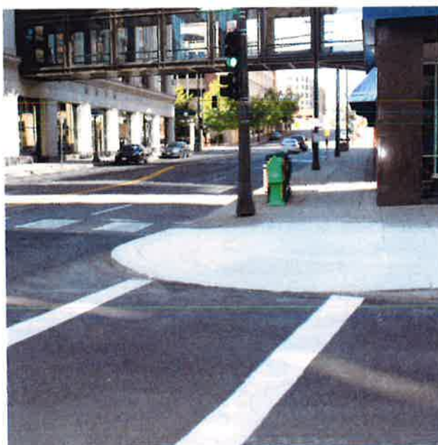
Tighter curb radii are particularly appropriate in downtown Main Street contexts.
