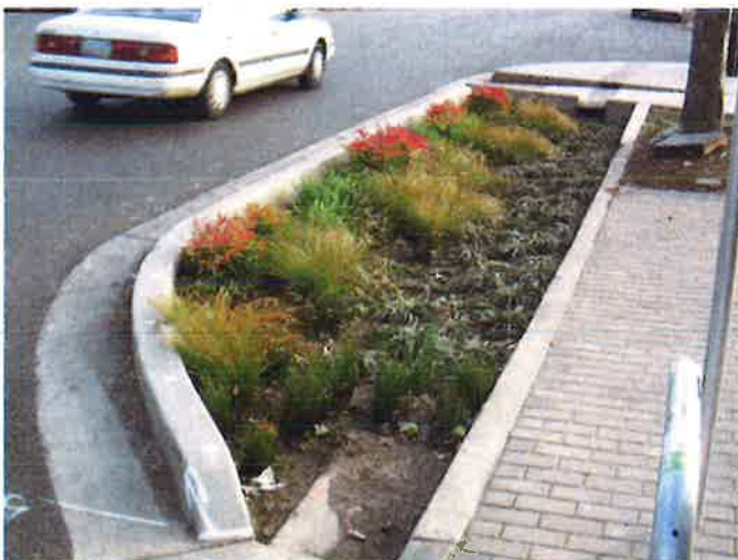
LID bulbout stormwater planter
