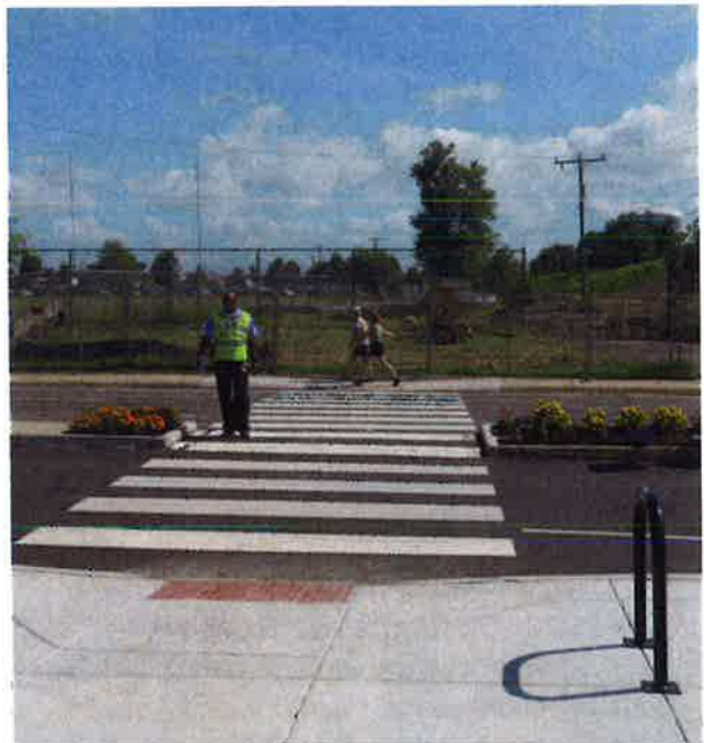
Crossing islands enable pedestrians to cross the street in two stages.
