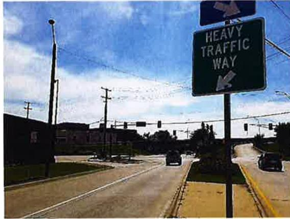
In this location, a 54-foot cartpath holds four driving lanes, should be restriped as *Street Type 54-BDDDDDB*: four driving lanes flanked by two 6-foot bike lanes. At Houston Avenue, bright paint should be applied to mark the bike lane turn onto Houston. Where there is a median for a 50-foot long stretch, the section should be restriped as *Street Type 54-BDDMDDDB*: the bike lanes must drop to 4 feet in width.
